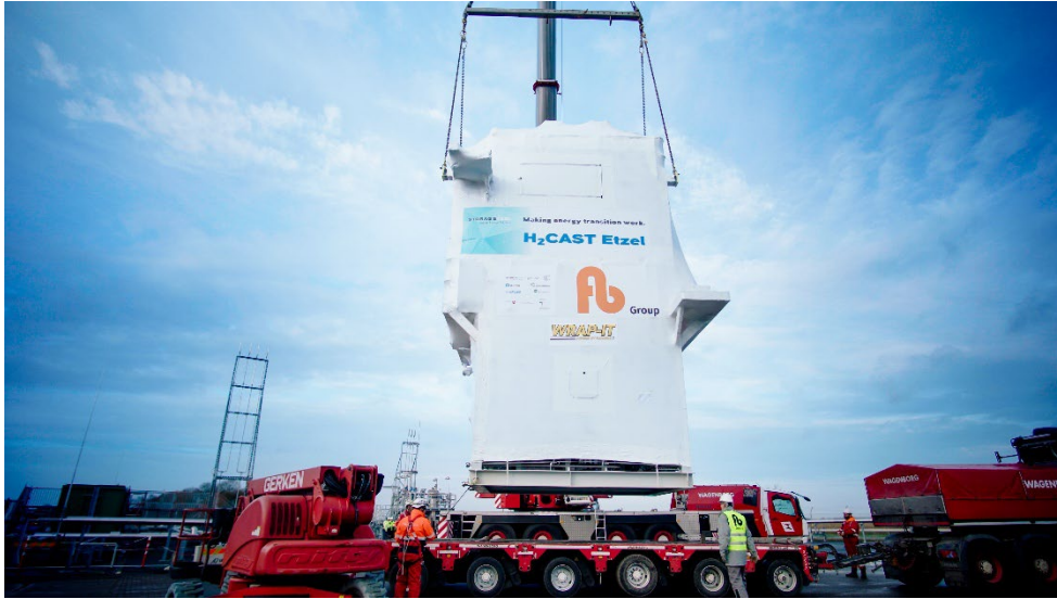
Fig.: The larger of the two components is unloaded at the H2CAST cavern site using a heavy-duty crane (Source: STORAG ETZEL / Gasunie)
